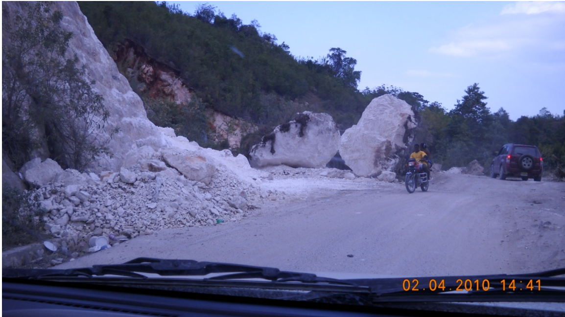
Figure 9.8 Topple or fall included several large boulders in this old quarry. (N18.439010, W72.646168).
