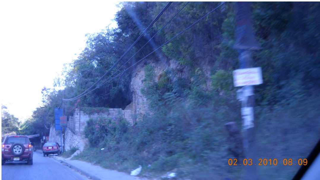
Figure 9.6 Stable near-vertical road cut and masonry wall. (N18.531873, W72.313045).
